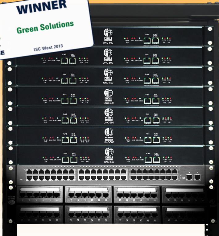
UNC-500-FT-8R-RM Shown in multiple controller rack
