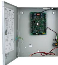
NIRC-2000-UL includes one NIRC-2000-B controller installed in an ENCL-1-PS enclosure with tamper switch
